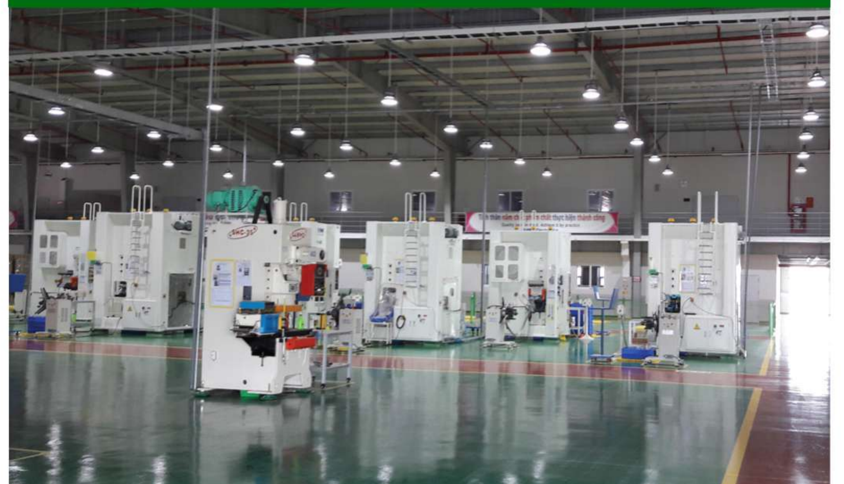
Installing power and water system
